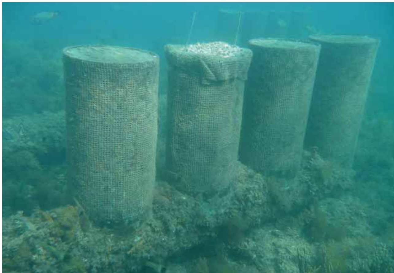
PLATE 11-1 YUMBAH SEAWATER INTAKES (RISERS) IN SMITH BAY
