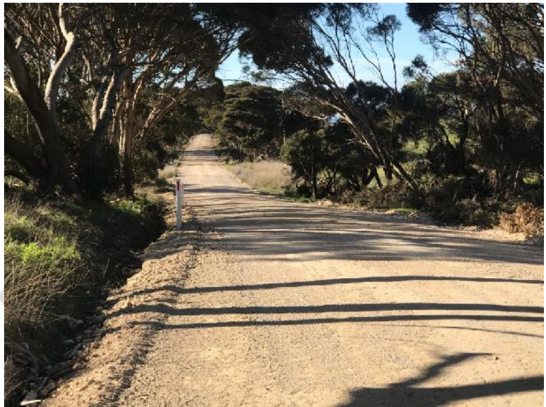
Gap Road 2 - typical standard between Springs Road and North Coast Road
