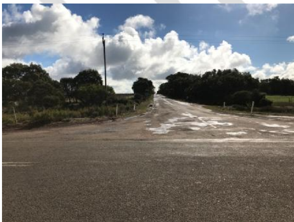
Stokes Bay Road 5 - intersection with Playford Highway
