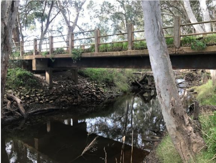
Ropers Road 3 - single lane bridge spanning Cygnet River
