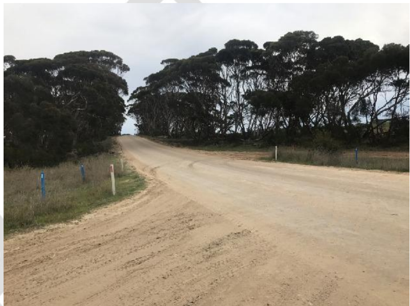
North Coast Road 5 - intersection with Gap Road
