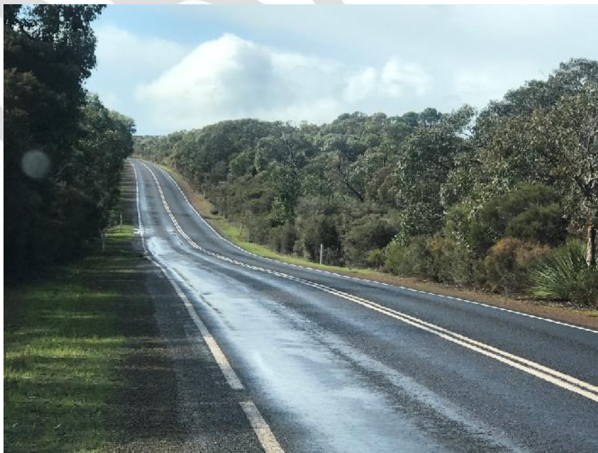
Playford Highway 6 - typical condition
