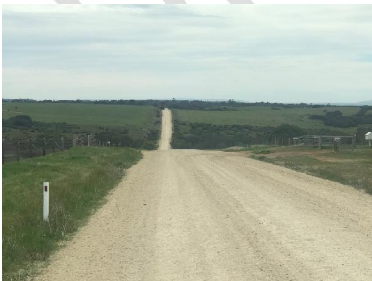
Springs Road 1 – at Woodlana looking east
