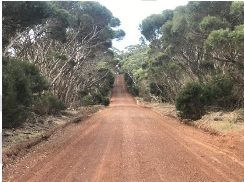
Gap Road 1 - typical condition
