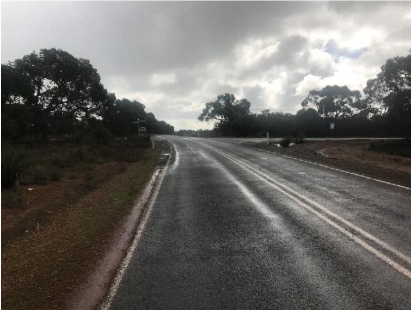
Stokes Bay Road 4 - intersection with Weatheralls & Morgans Roads
