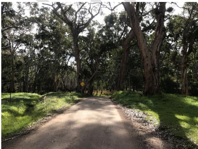
Ropers Road 2 - approaching floodway section that would require to be built up with substantial tree removal
