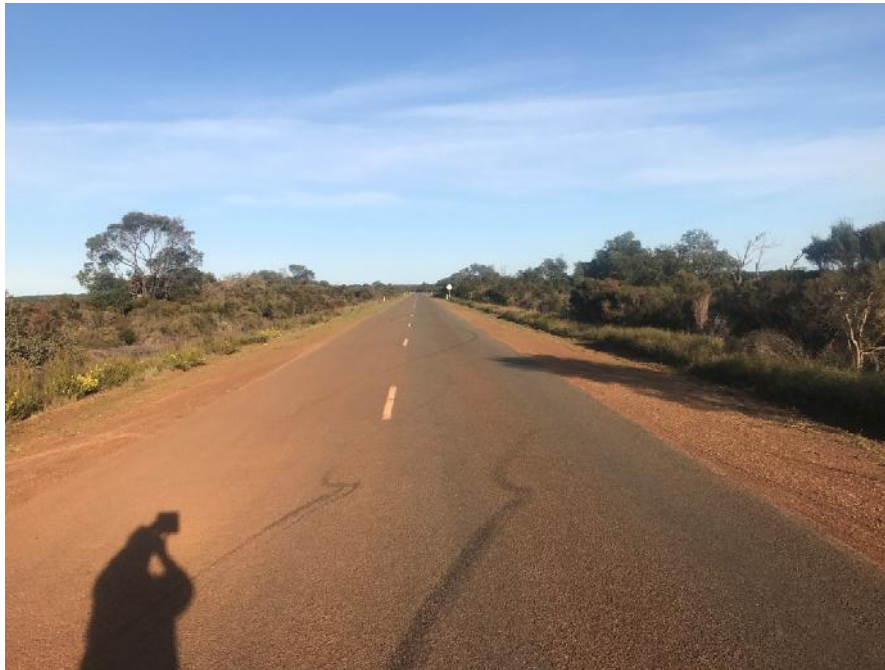
Playford Highway A 1 - typical condition and clearances
