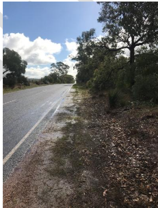
Stokes Bay Road 3- roadside vegetation
