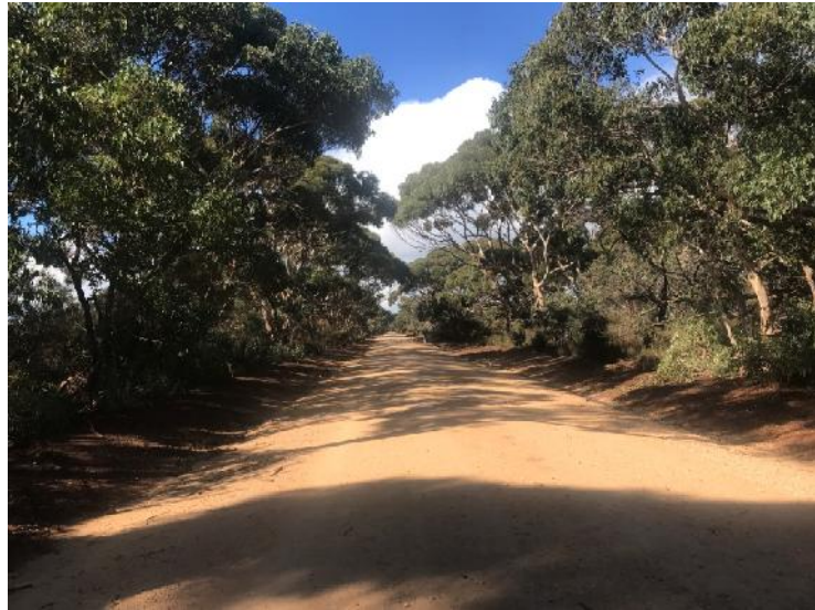
Bark Hut Road 1 - typical condition
