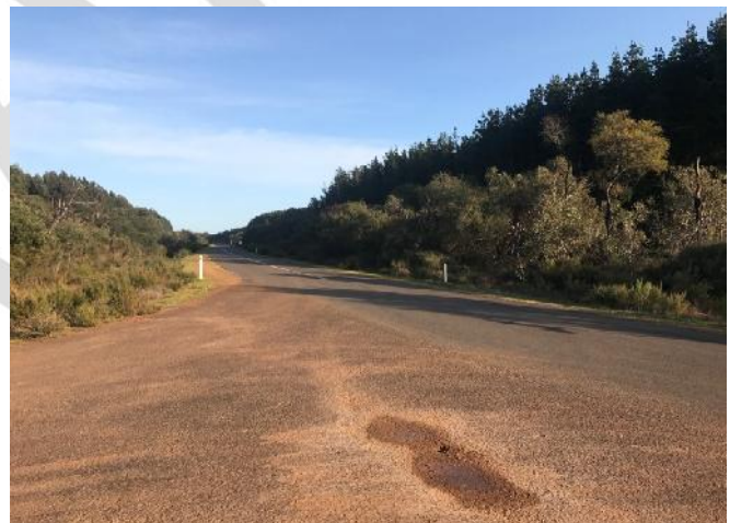
Playford Highway A 3 - Mt Taylor Road intersection (looking west)
