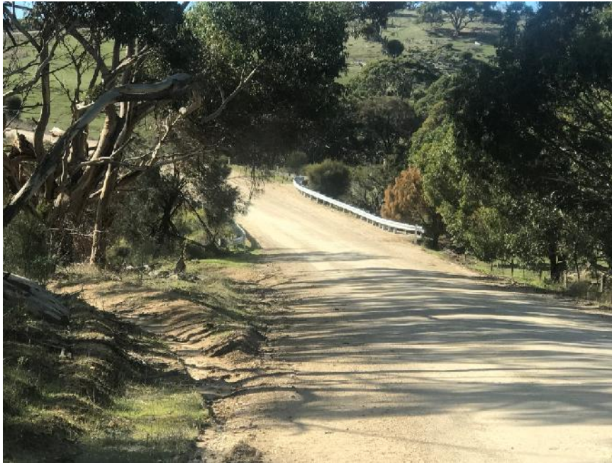
North Coast Road 2 – approaching bridge
