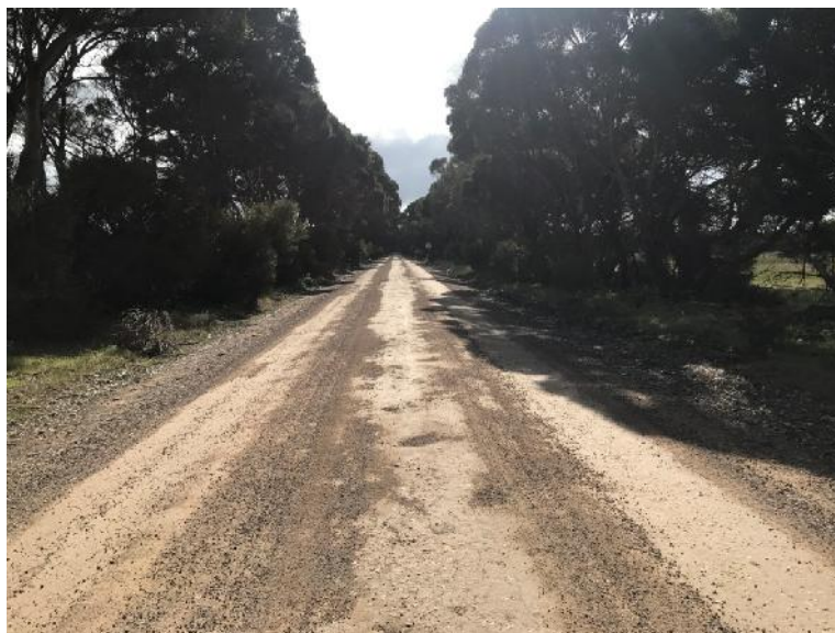
Ropers Road 1 – typical standard (200m off Playford Highway)
