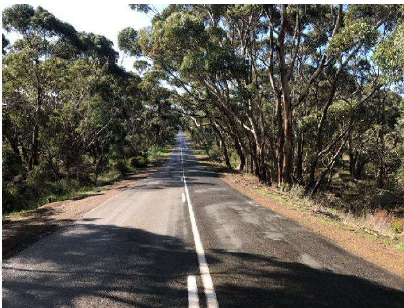
Playford Highway 5 – section east of Bark Hut Road intersection subject to inundation during prolonged, heavy rain events.
