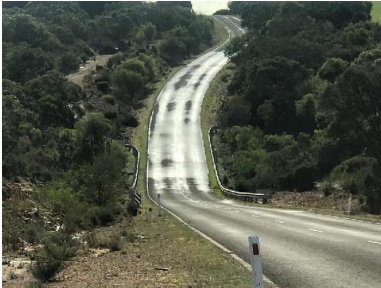
Stokes Bay Road 2 - bridge over Cygnet River
